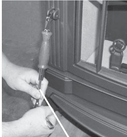
Secure using 7/16" socket wrench.
